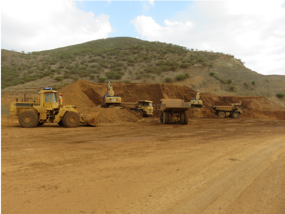
Figure 2: Stockpile reclamation prior to ship loading Tontouta (SMGM)
