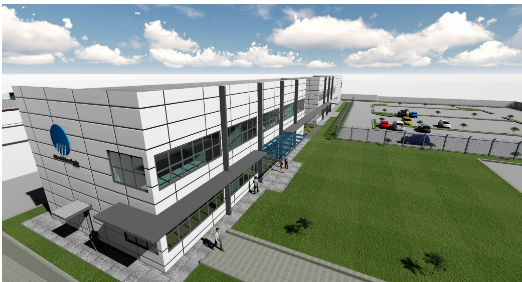
Figure 3 – Administration and Process Building
