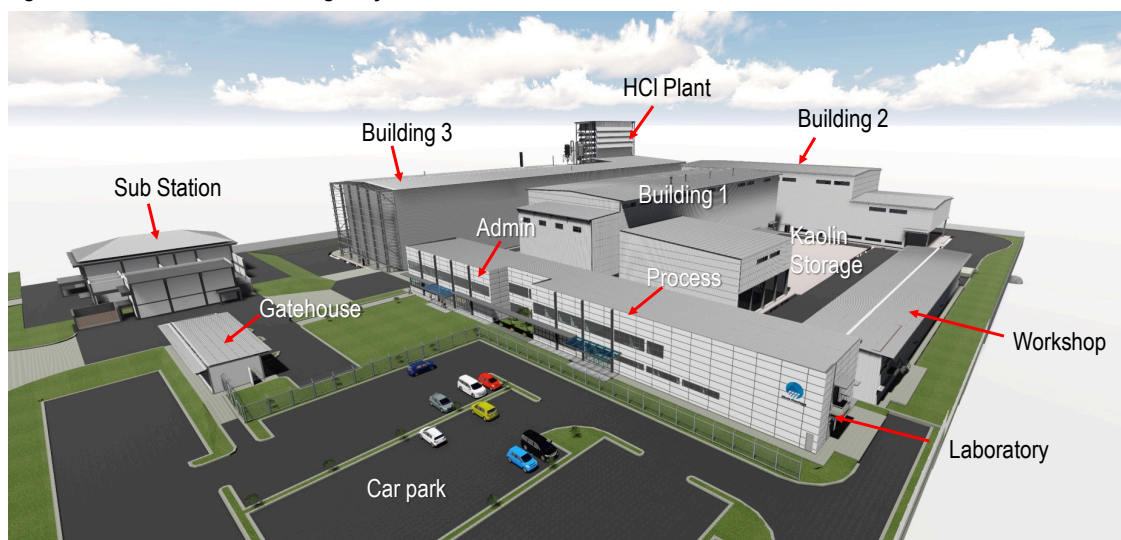
Figure 1 – HPA Plant Final Buildings Layout
