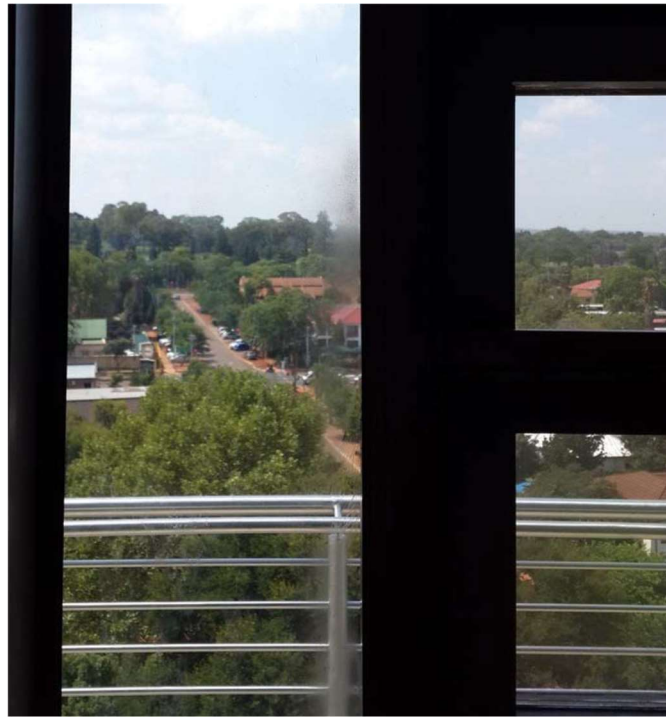
Installed solar façade, six 200x200mm panels – Standard glass on the left Transparent ClearVue window placed in front of glass façade on the right
