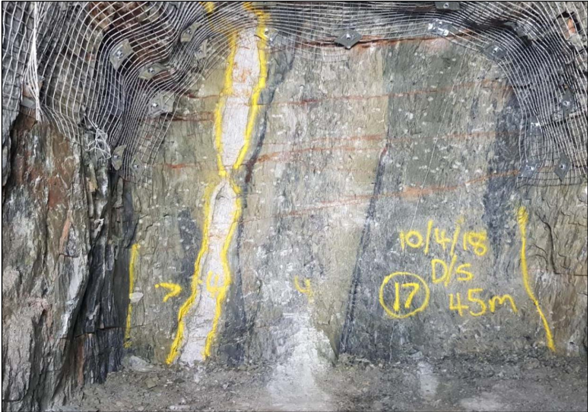
Figure 2: Level 2 North Ore Drive at 10 April 2018.
