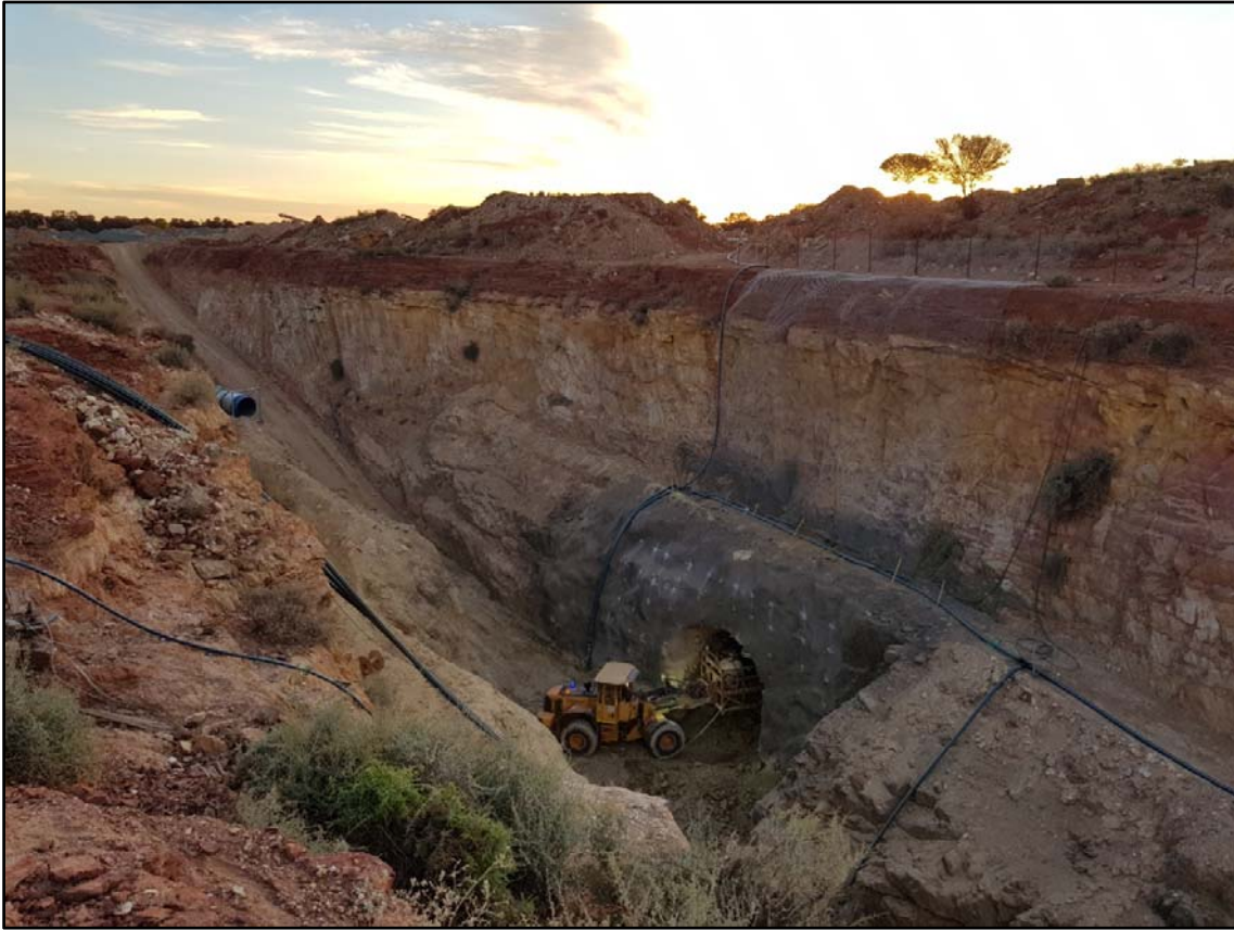
Figure 4: Charging the portal opening.
