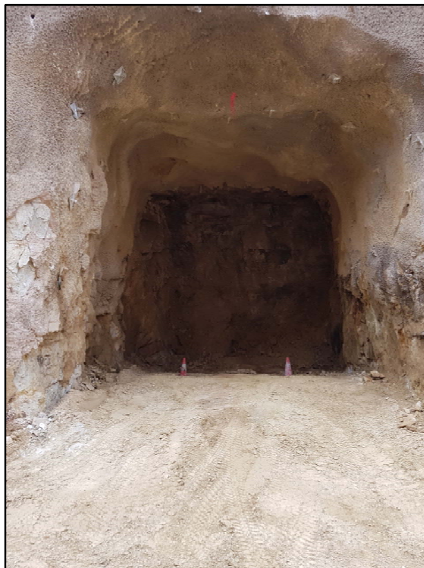
Figure 3: Mine portal opening after completion of boggging.
