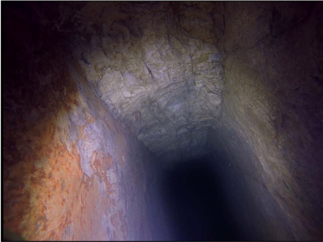
Figure 7: Underwater drone survey - Main Vein exposed in crown pillar of the Level 1 stopes (width approximately 0.75m wide).
