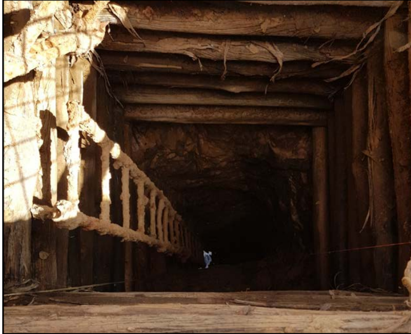
Figure 4: Photograph looking down historic North Shaft at the Second Fortune Deposit
