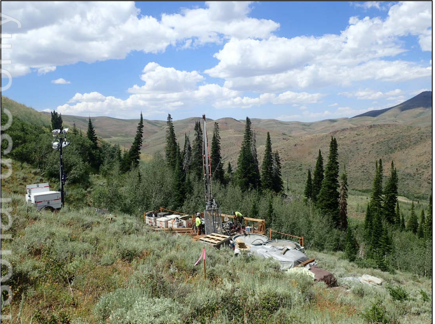
Image 2: Drill rig at the Big Springs Project
