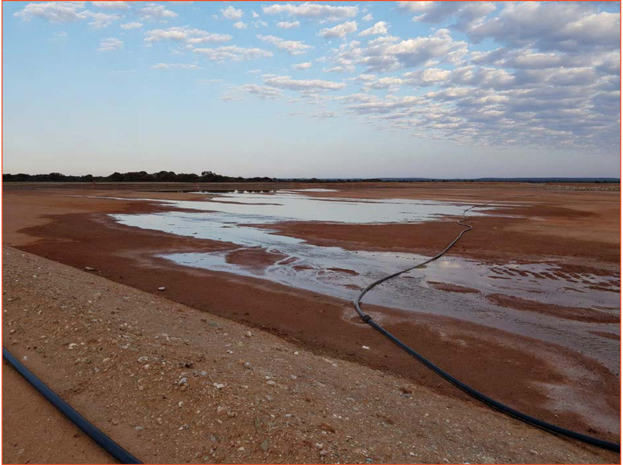
Image 2: Evaporation ponds in use
