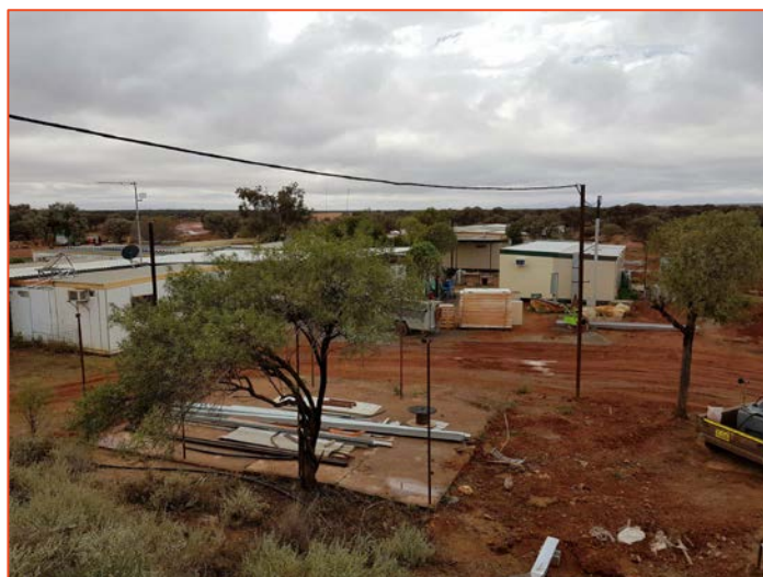
Image 1: Camp development work underway
