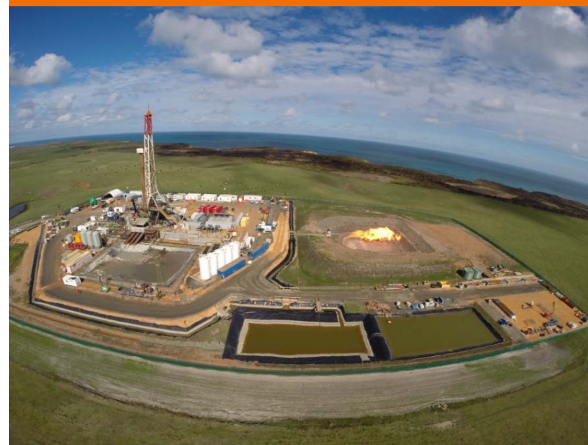
Aerial view of Halladale/Speculant well site
