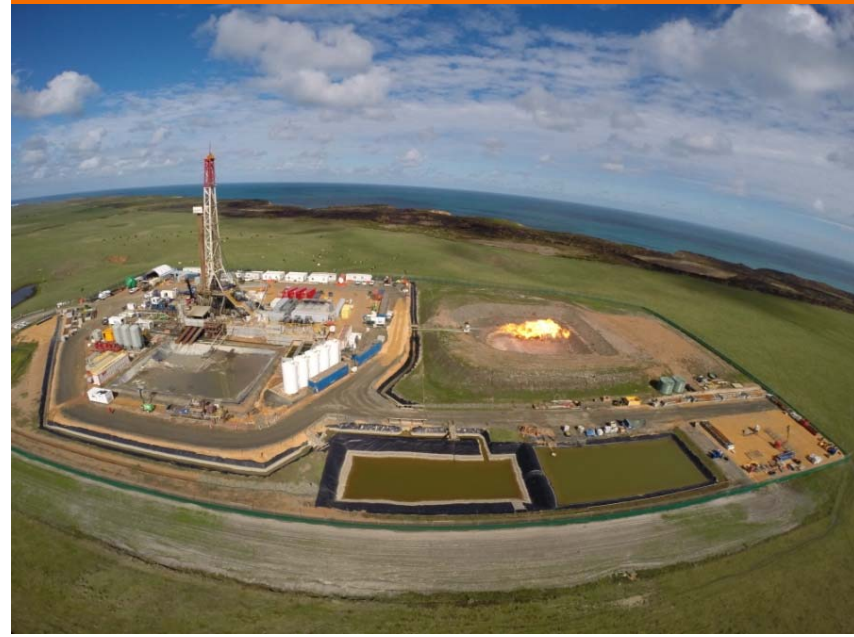
Aerial view of Halladale/Speculant well site
