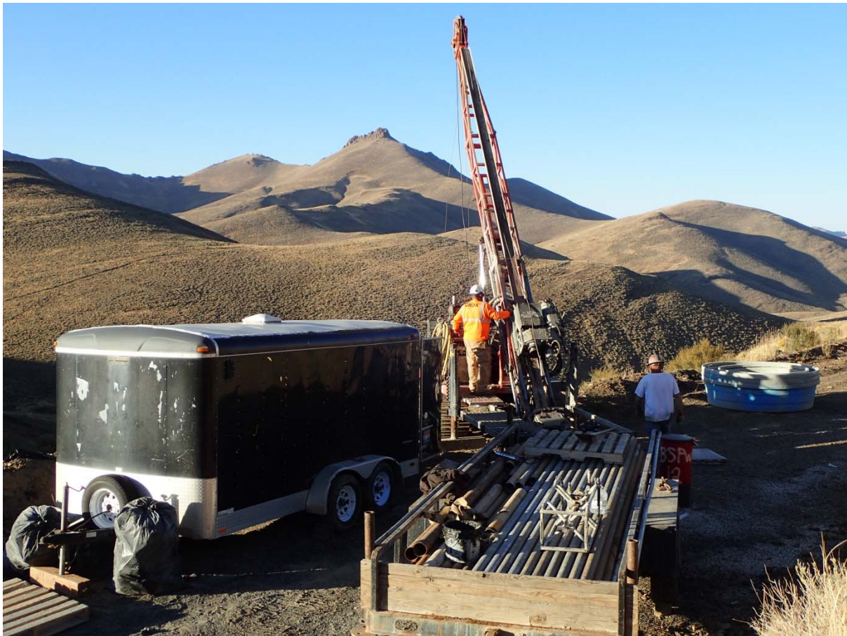
Image 1: Geotechnical drilling at North Sammy - Big Springs Project, Nevada.
