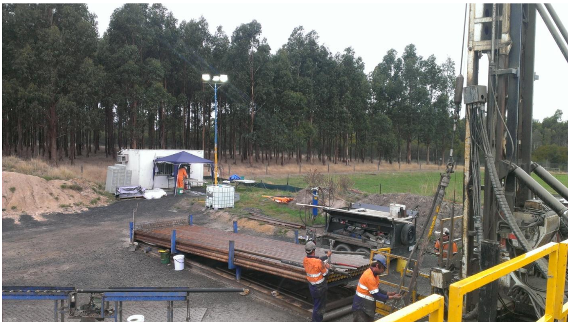
Yallourn Power 1: view from rig towards core lab set- up
