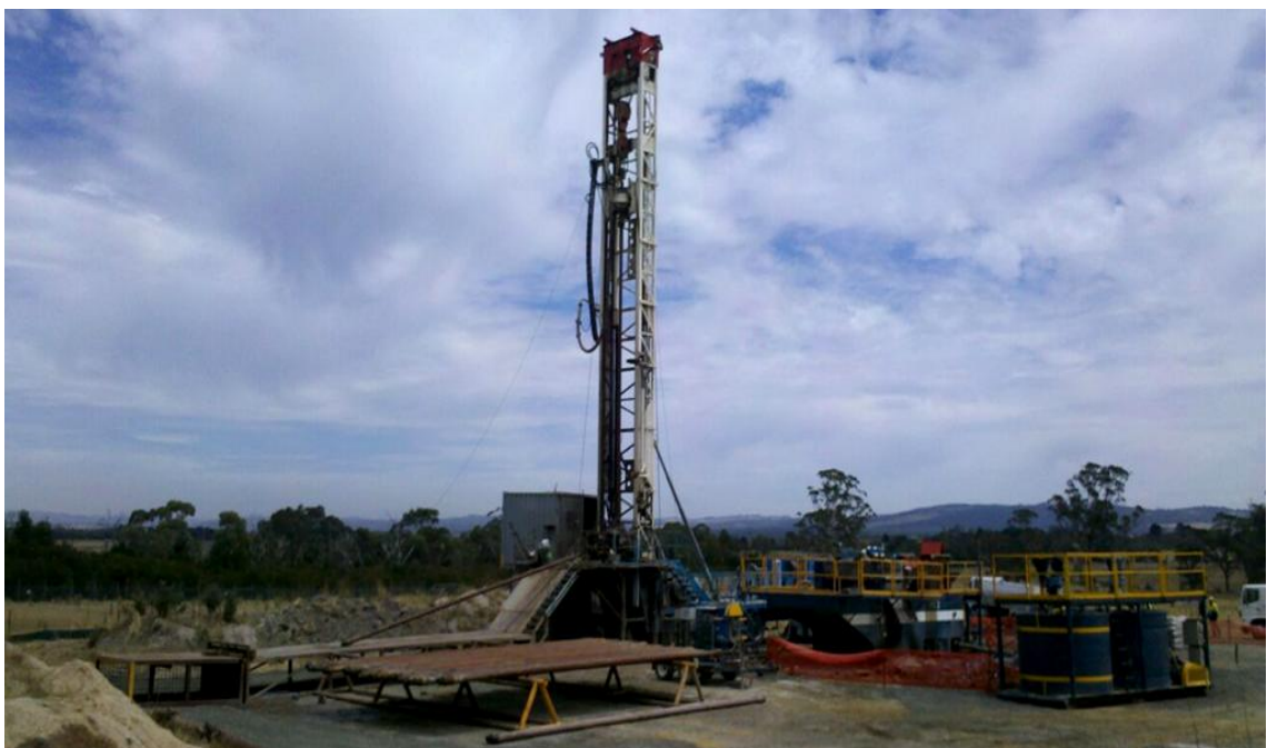
Yallourn Power 1 with the top hole rig on site
