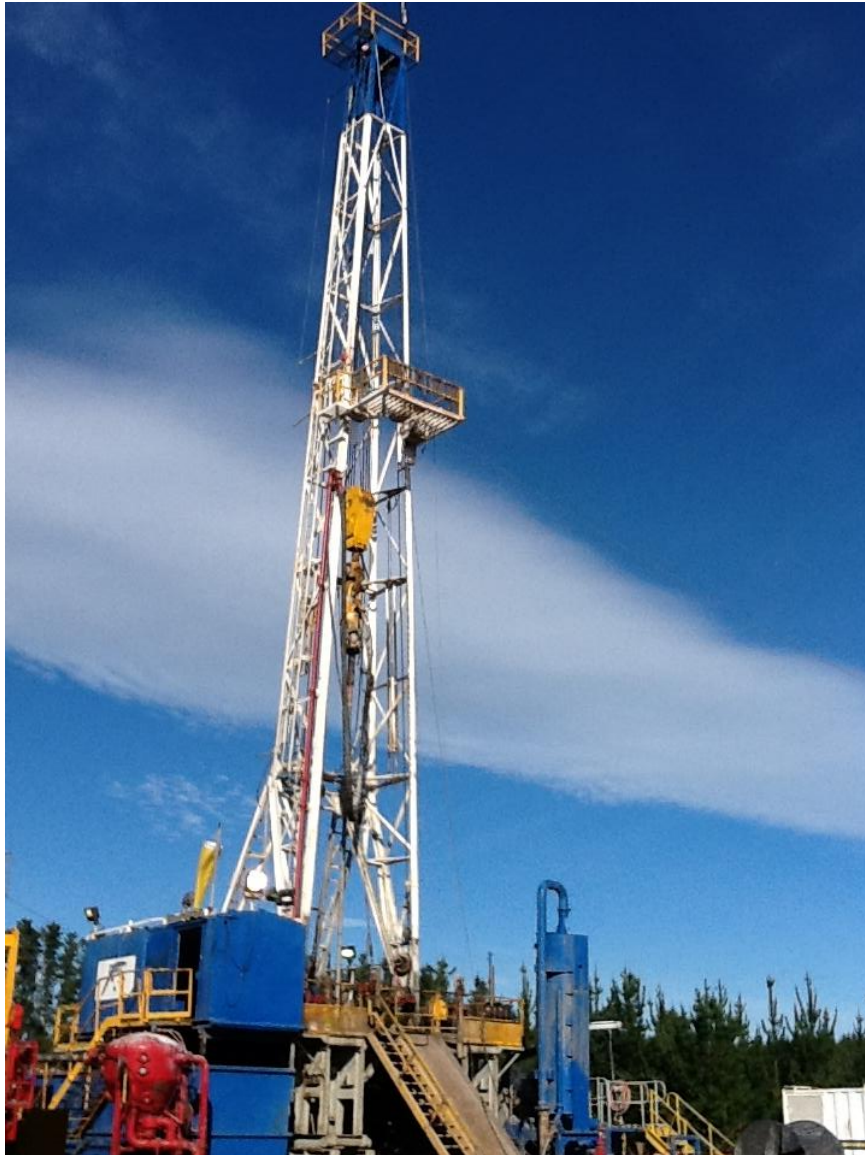
Holdgate 1: rig on site
