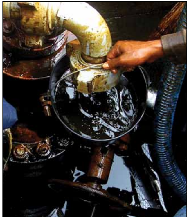
Figure 5 - Oil produced from Malolos-1 after 'nitrogen enhancement'
