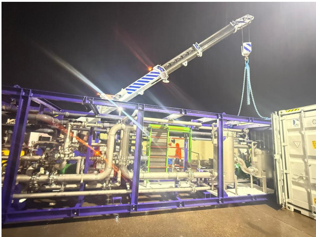
Figure 2. Load out of nano-filtration plant
