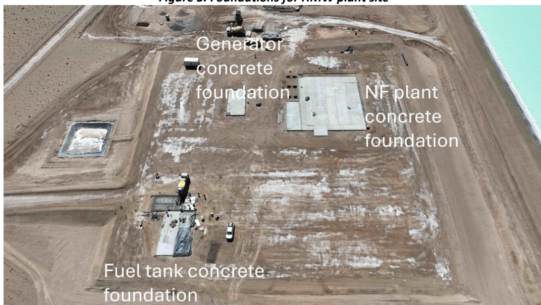
Figure 5. Foundations for HMW plant site
