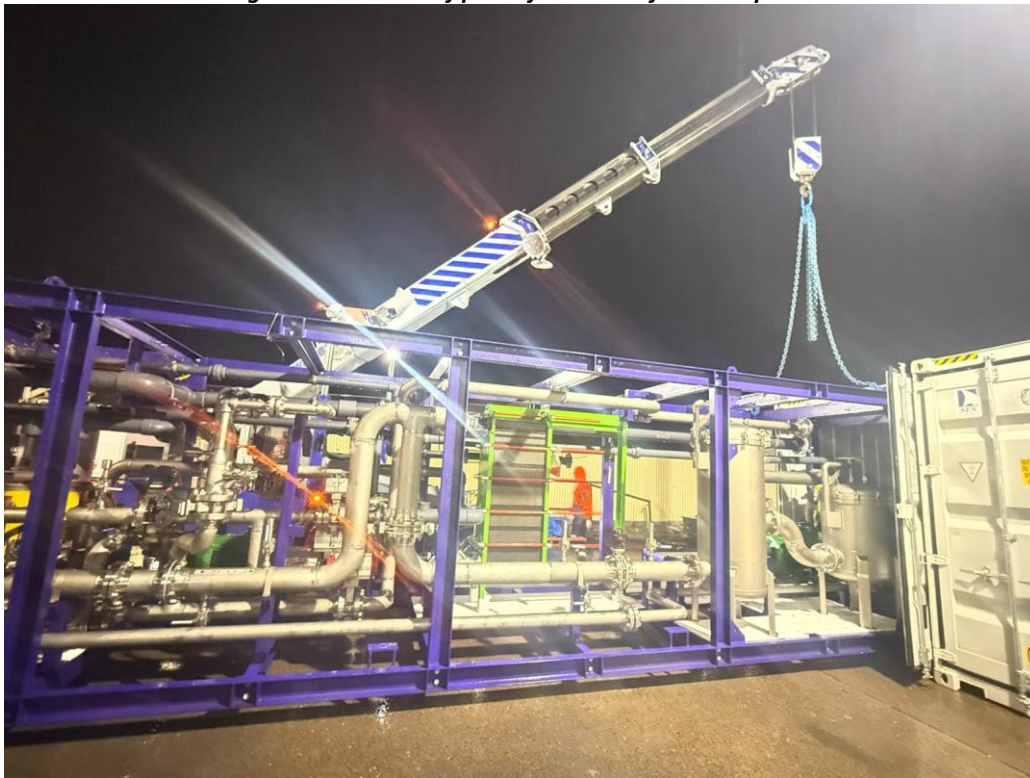
Figure 1. Load out of part of the nano-filtration plant
