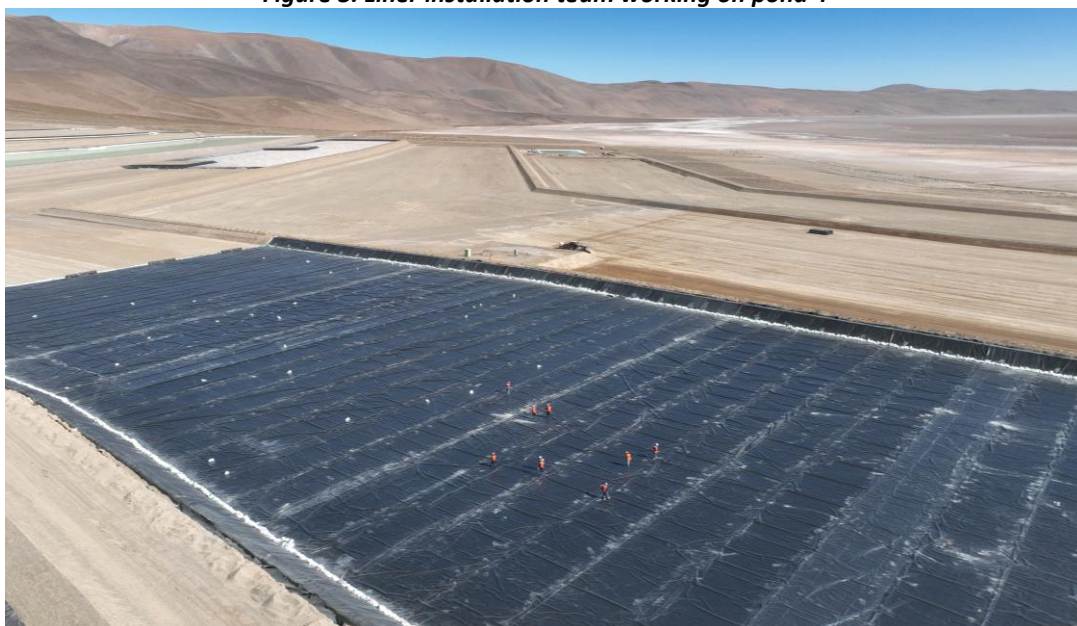
Figure 3. Liner installation team working on pond 4
