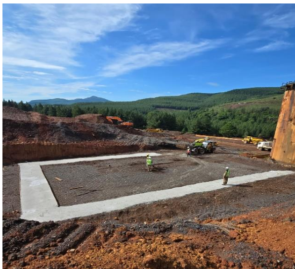
Figure 2: Blinding of the Gold Room's Foundations
