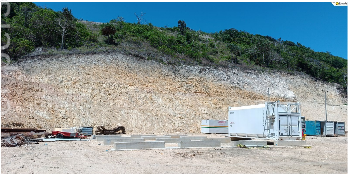
Image 2: Fuel storage foundations have been completed.
