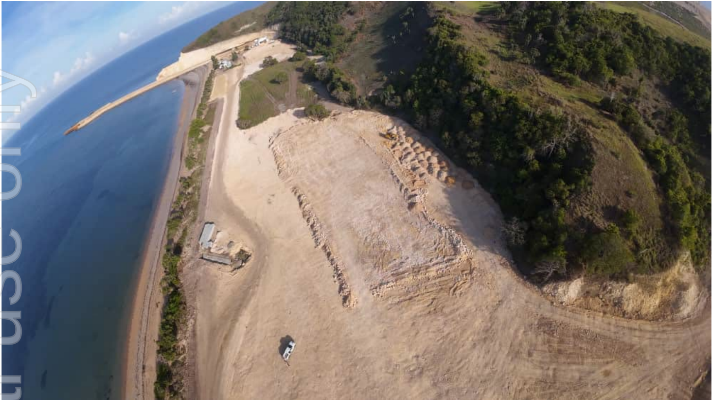
Image 9: Aerial shot of the bulk earthworks site preparation.
