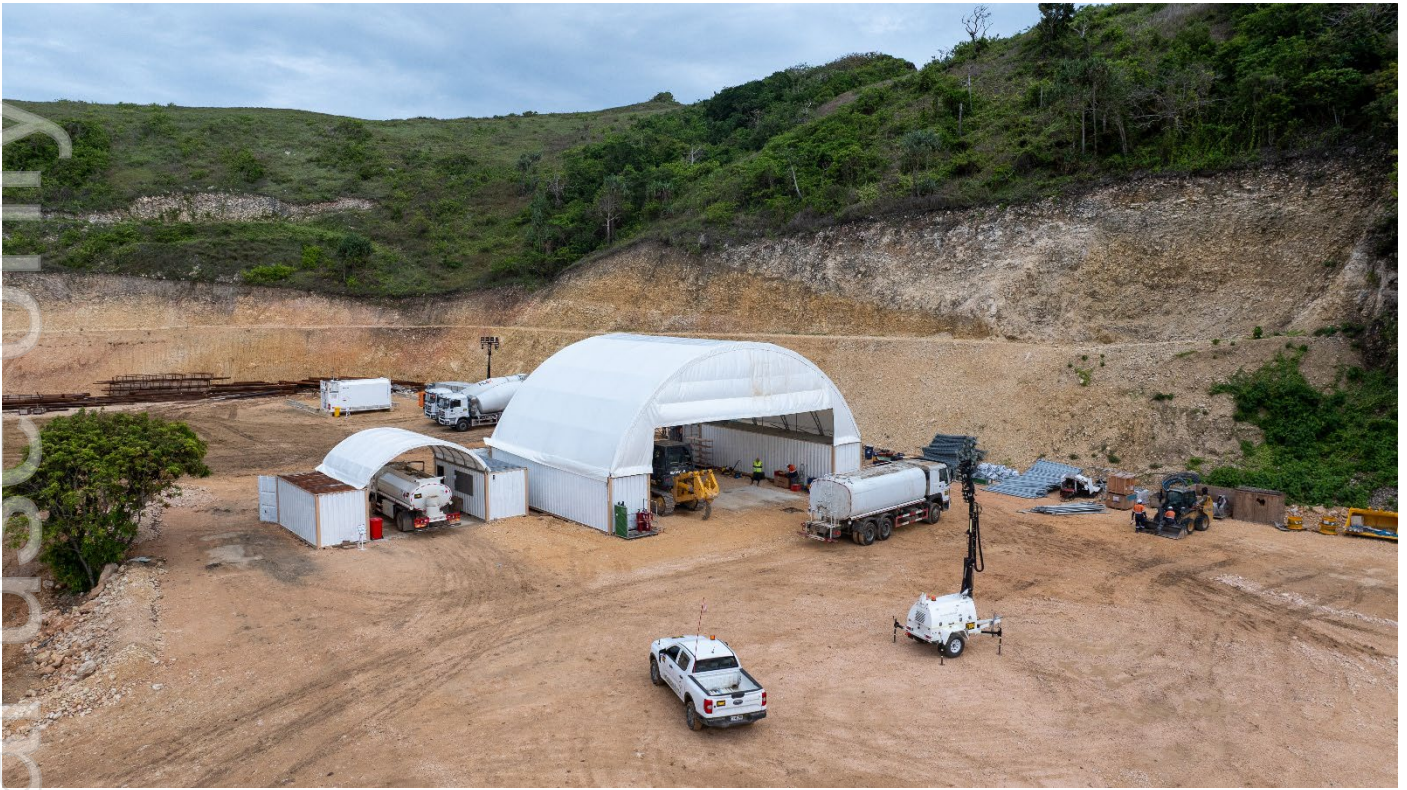
Image 5: Maintenance workshop completed and in use.
