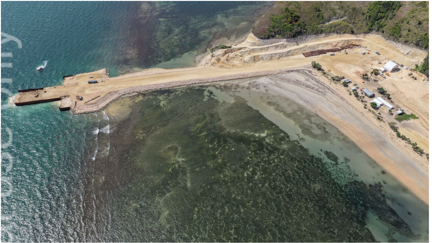
Image 3: Wharf construction is continuing.
