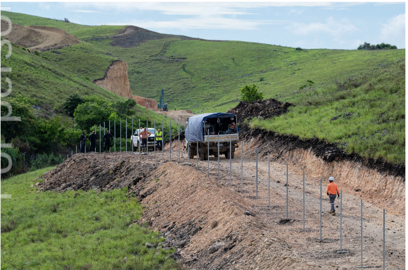
Image 4: Access Road Construction progressing, and fencing of the Mining Lease area.
