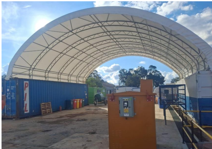
IMAGE 4: TEMPORARY WORKSHOP BOOSTING MAINTENANCE READINESS AS DEVELOPMENT ADVANCES
