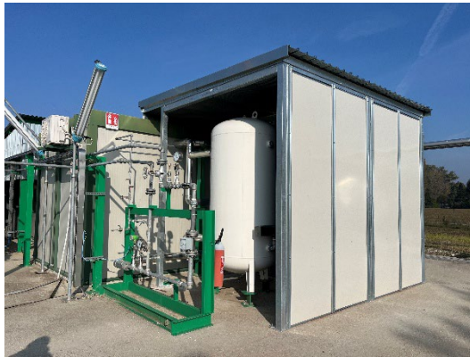
Image 1 – Sound insulation barriers
