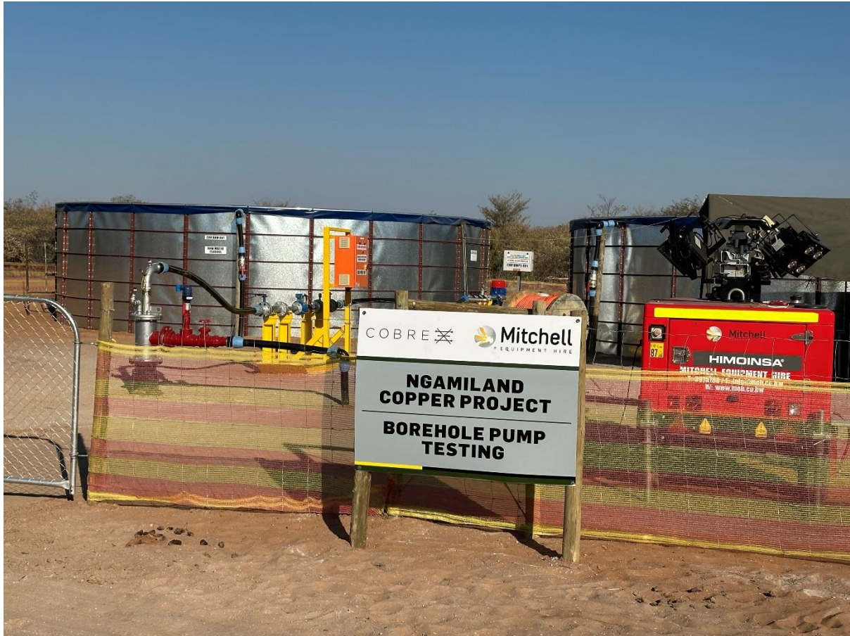
Figure 2. Hydrogeological pump and injection testing, NCP Botswana
