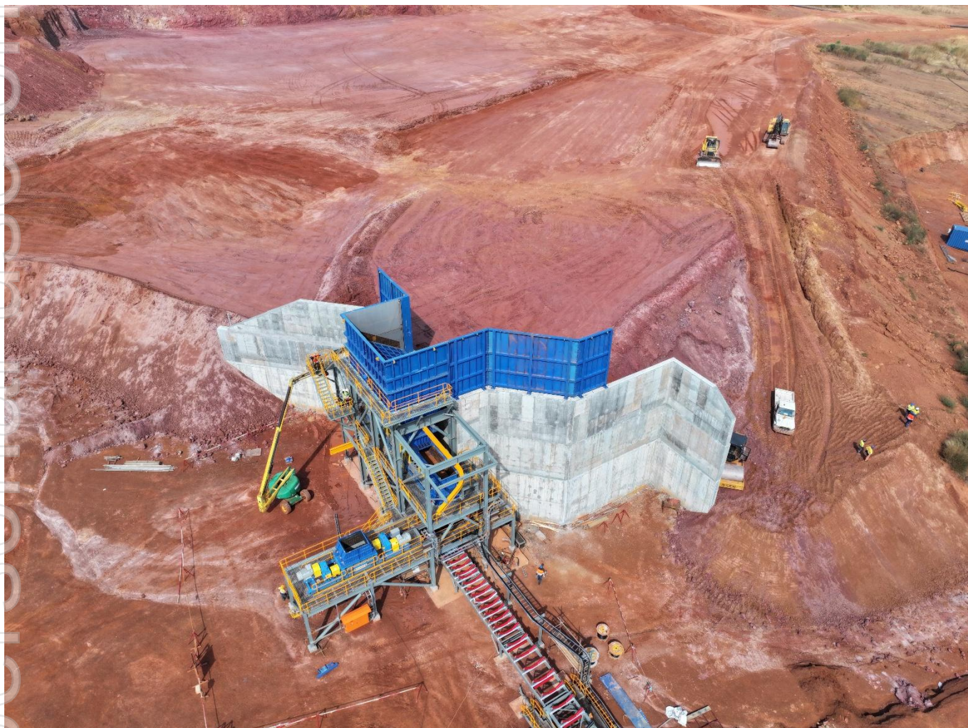
Figure 2: Saprolite crushing plant (15 November 2025)
