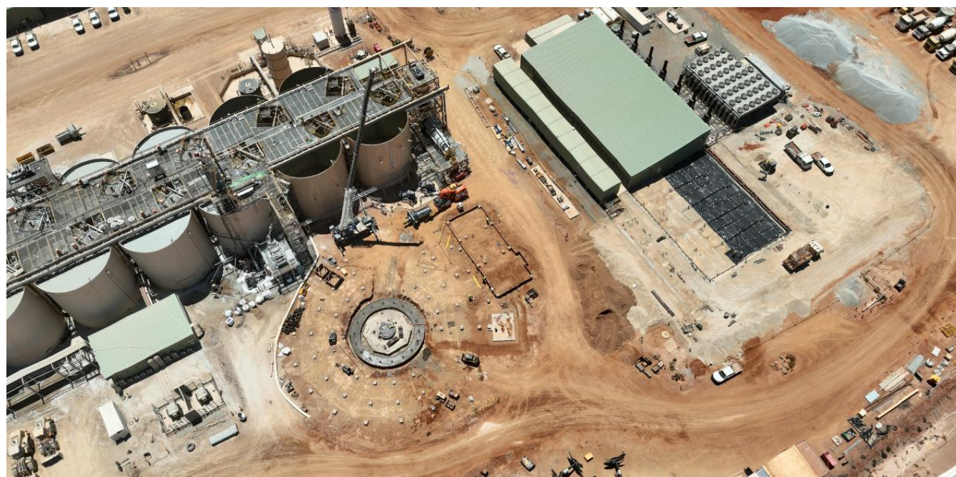
Wet plant & power station
