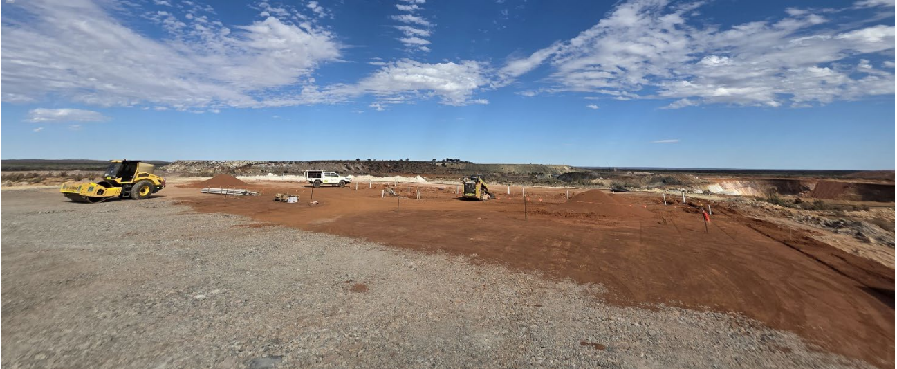
Figure 3 – Preparation for site offices and workshops advancing
