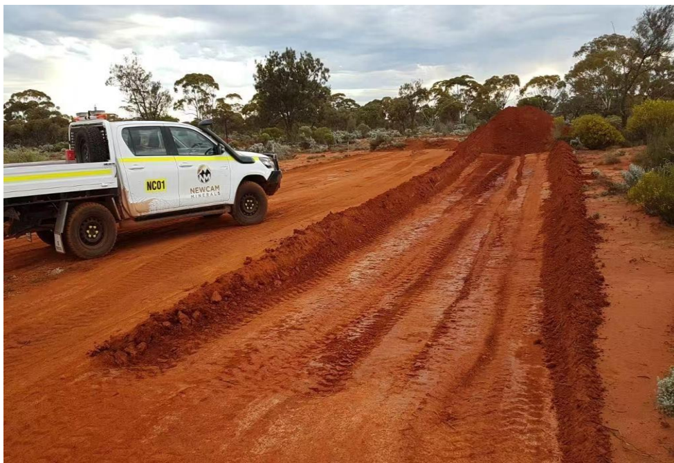
Figure 6: Drill pad clearing and earthwork in progress at Gimlet
