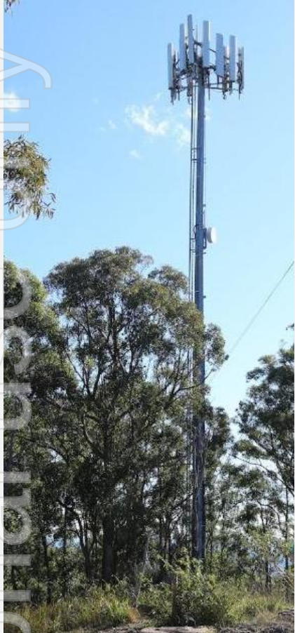
Securing mobile tower access
