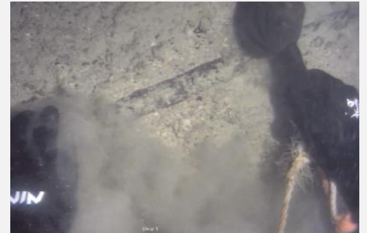
Monitoring of subsea telco cables
