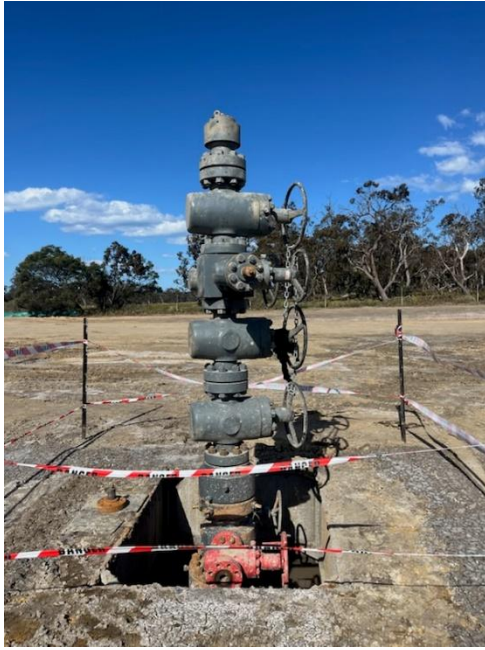
Figure 2: Wombat-5 wellhead installation
