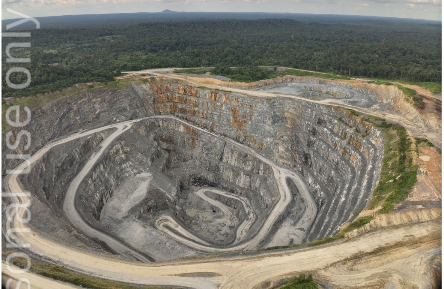
Figure 1 | Okvau Open Pit – October 2025
