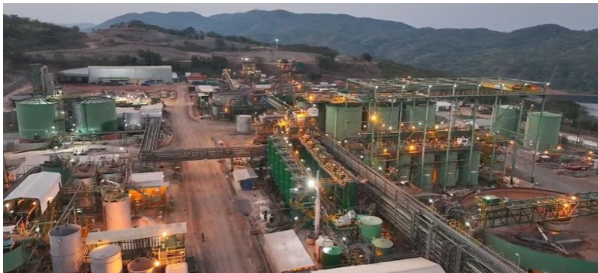
Figure 5: Leaching, RIP, elution and precipitation circuits
