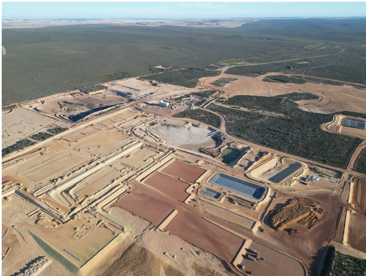
Picture 5. Iluka's Eneabba Rare Earths Refinery, Western Australia.
