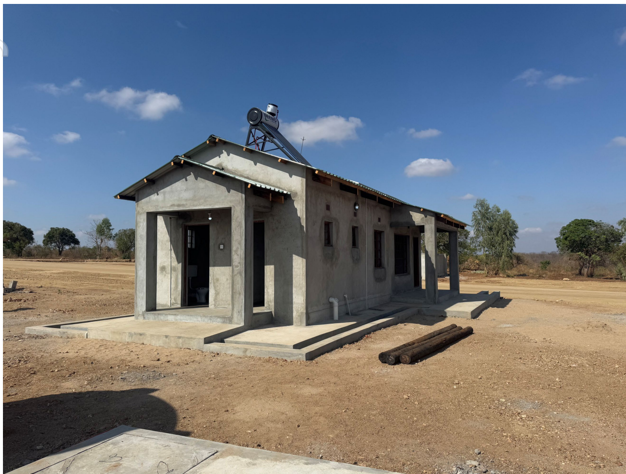
Picture 2. Security building on site at Kangankunde.
