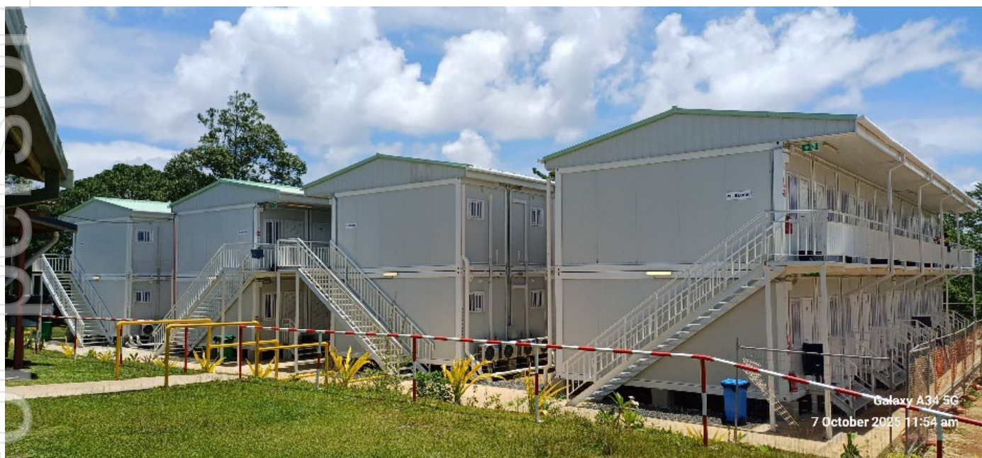
Figure 1. Simberi Camp Expansion – New Accommodation Buildings
