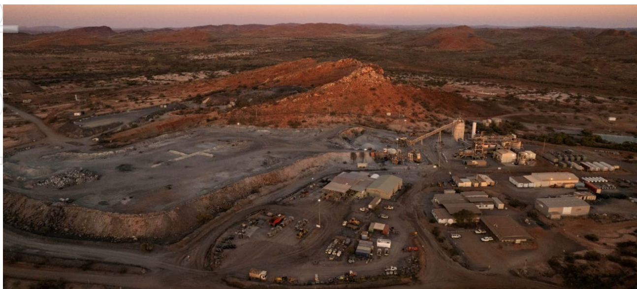
Figure 1: Paulsens mine site, September 2025.
