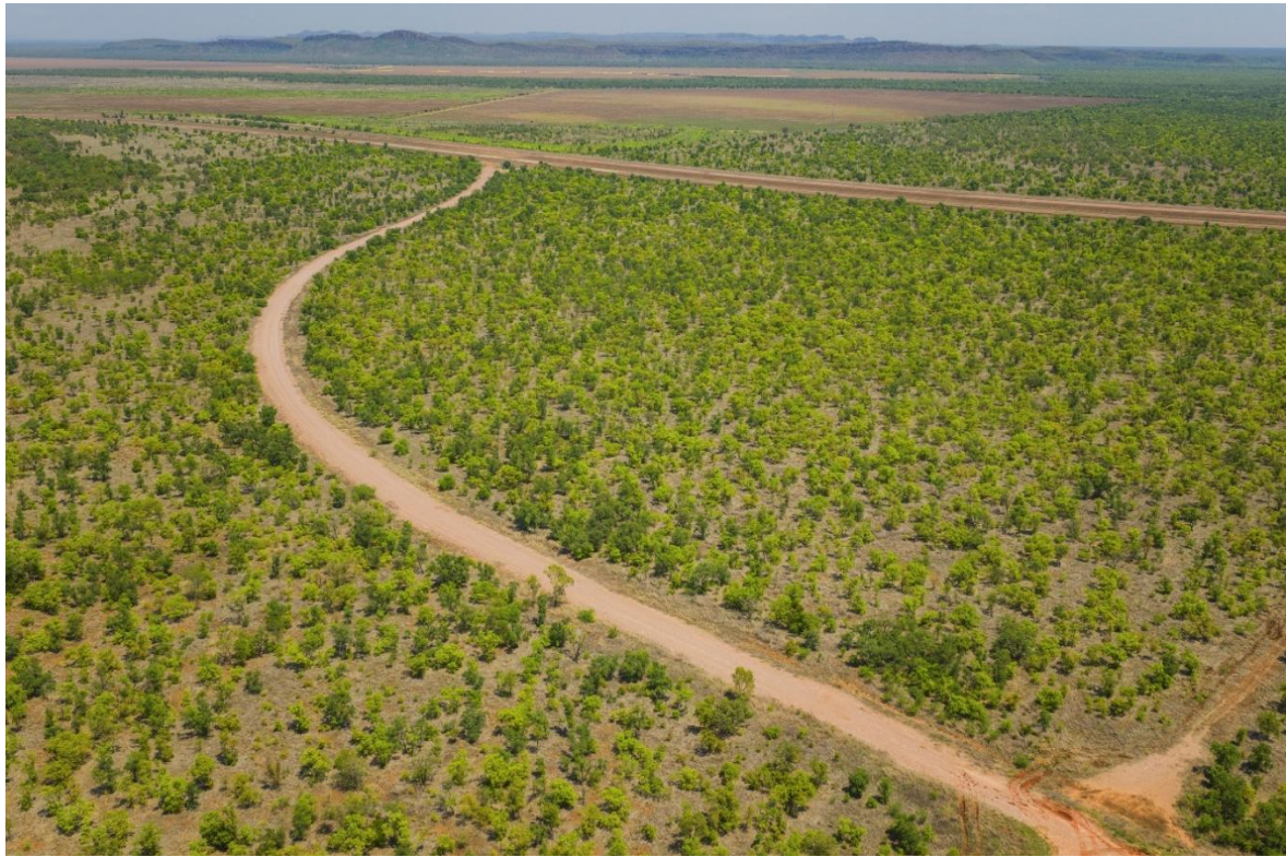
Figure: Internal Access Road
