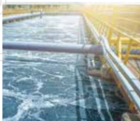
Wastewater treatment plant
