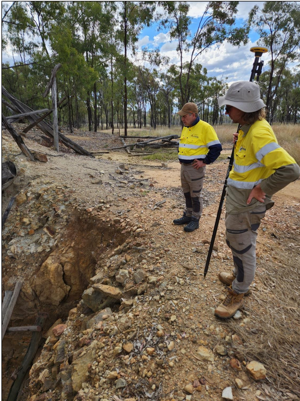
Figure 5: James Chirnside Dart Mining Chairman (left) and geologist Riley Jenkins inspecting the Historic Banshee shaft and collapsed Crown Pillar.
