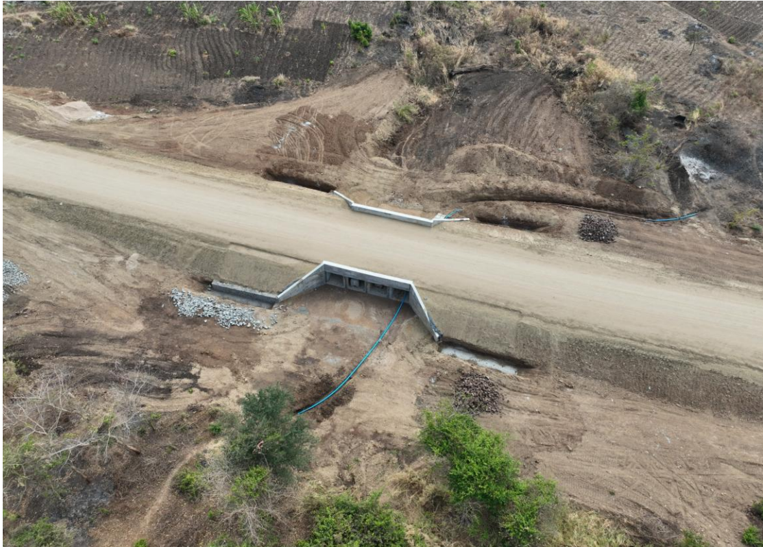
Picture 1. Completed culvert on site at Kangankunde.
