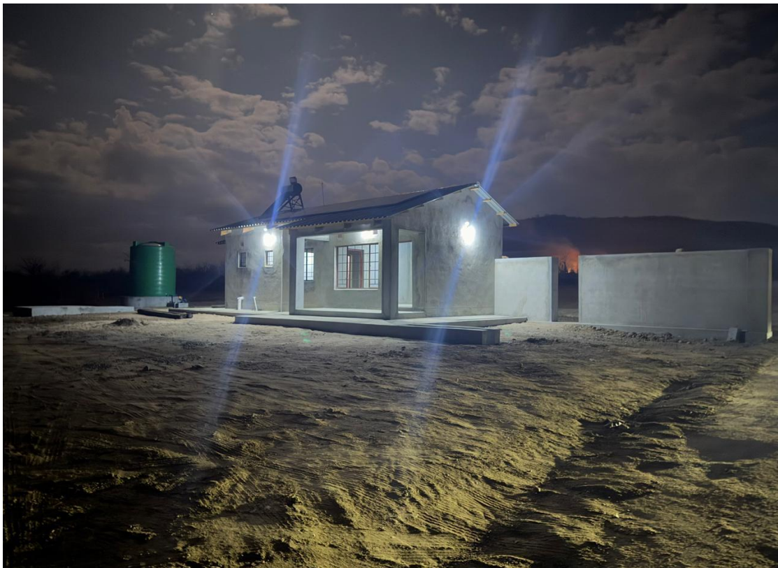
Picture 2. Security building at Kangankunde.
