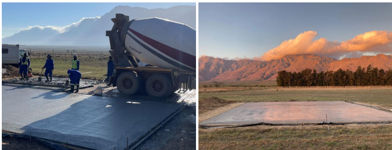
Figure 1: Pouring of the slab at Bontebok Ridge Reserve in Wellington, South Africa and the slab undercover during curing.
