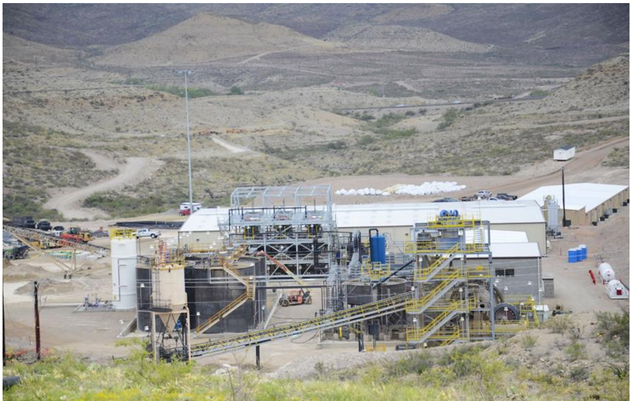
Figure 3: Shafter Processing Infrastructure.
