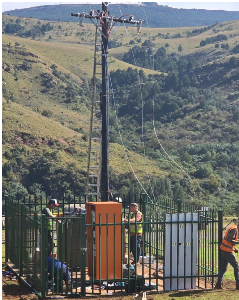
Figure 2: Installation of temporary electrical plant supply
