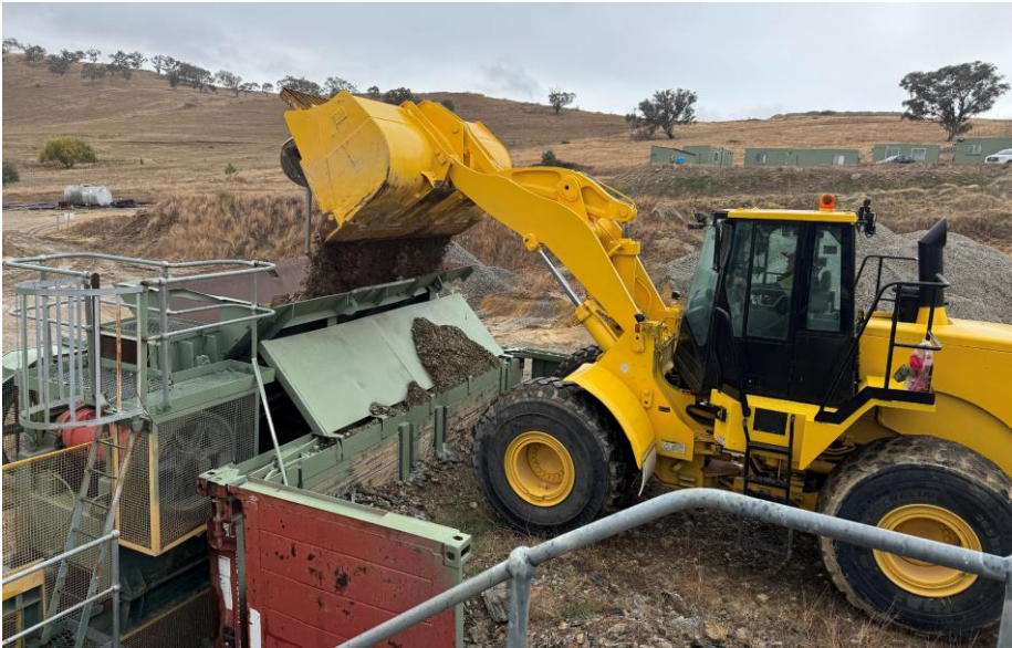
Figure F – Loader stacking high grade tailings on the Challenger ROM pad ready for feeding to the Gold Plant
