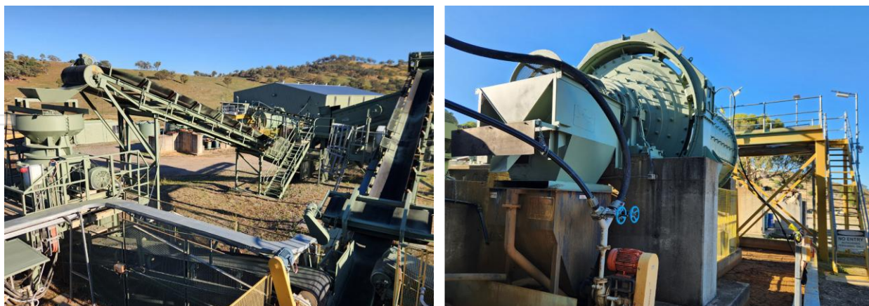
Figure D – The crushing and milling circuit at the Challenger Gold Mine has been repaired, tested, restarted and repainted. It is now operational.
