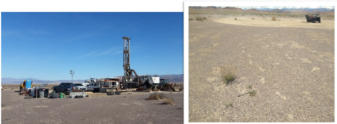
Figure 12. 2017 drilling operations shown above.
