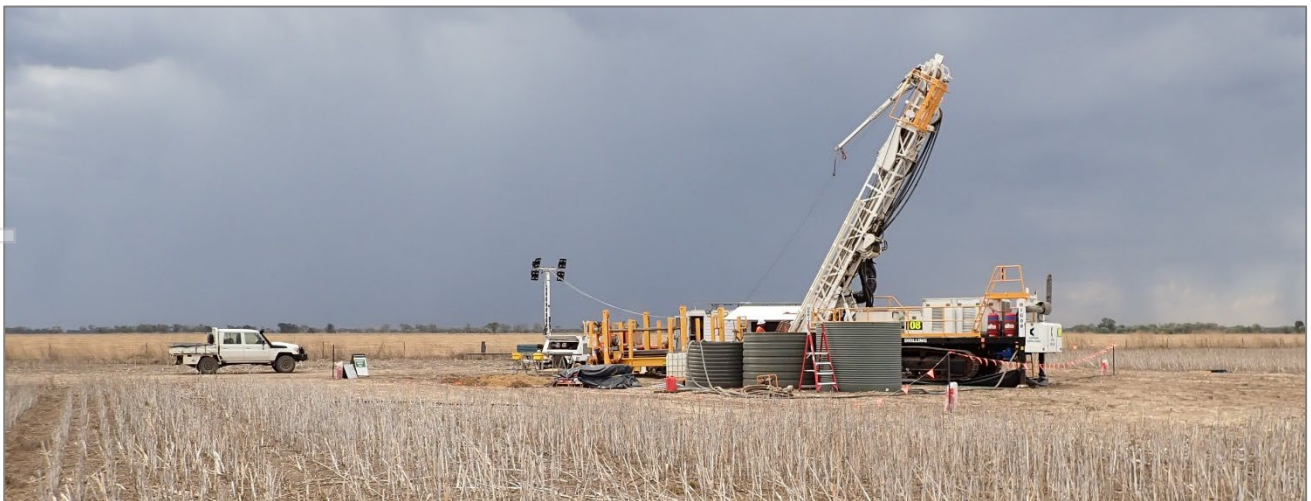
Figure 8. Drill rig on site at Corvette earlier in the year
