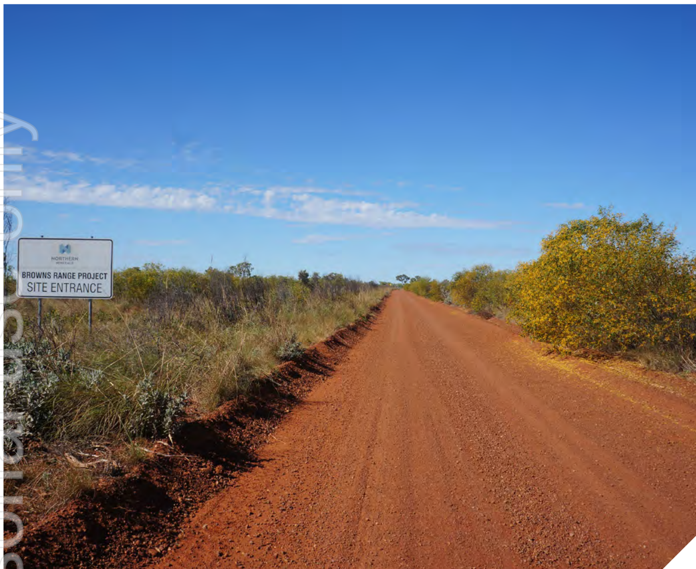
Figure 27 Existing site access road
