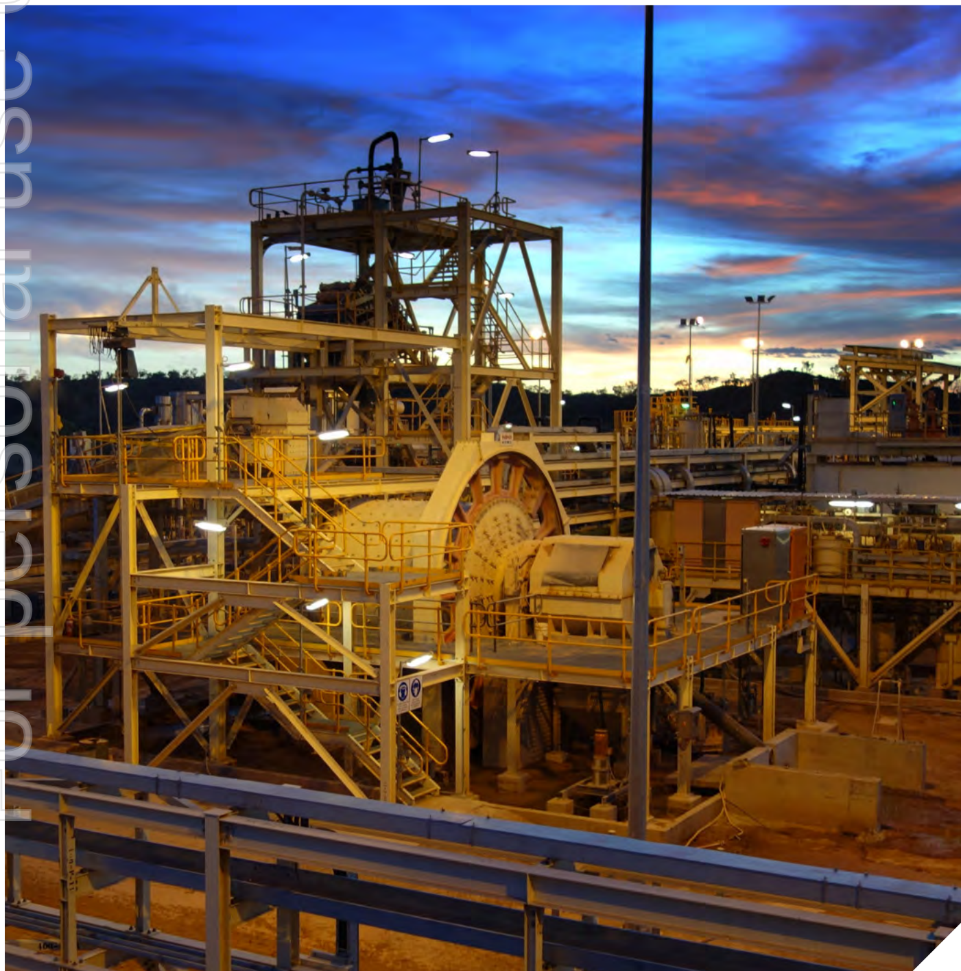
Figure 20 Browns Range Pilot Plant
