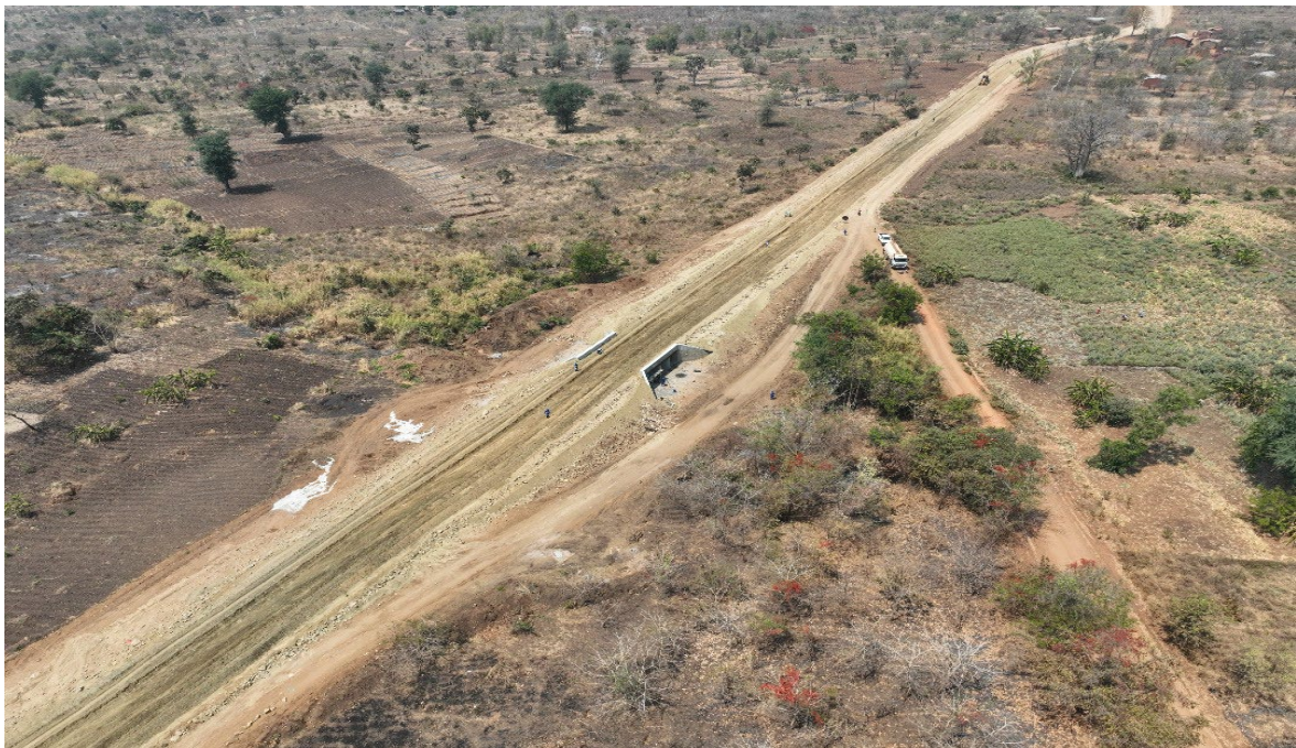
Picture 2 Access road to site with culvert installation complete.
