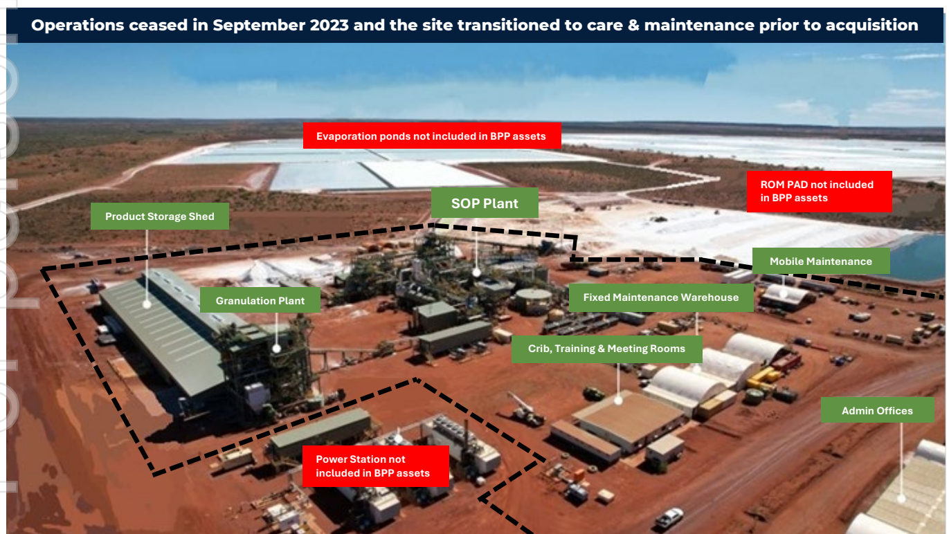
Figure 1 – Photograph of the Beyondie Potash Project in 2023 when in operation by KLL. The assets acquired comprise a fully constructed processing plant, site offices and maintenance infrastructure. Specific plant components include, KTMS crushing circuit, Kainite conversion circuit, column flotation circuit, liquor cooling heat exchangers, evaporative cooling circuit, product separation centrifuges, SOP recovery and granulation units, RO water plant and a bulk storage shed.
