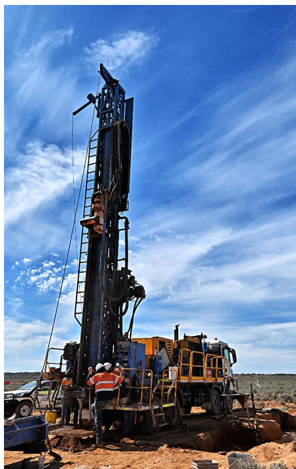
Figure 2 – Samphire ISR FRT production well drilling operations.
