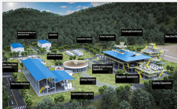
Kangankunde Processing Plant (Stage 1)
