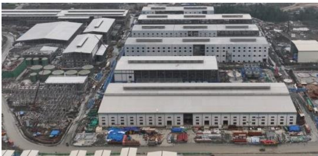
ENC integrated refinery construction progress
