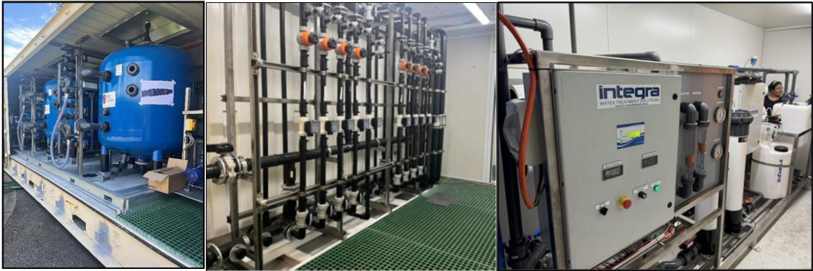
Figure 3 – Ion exchange module; Wellhouse (pipe room) module; Reverse Osmosis plant – currently situated in Alligators Whyalla yard
