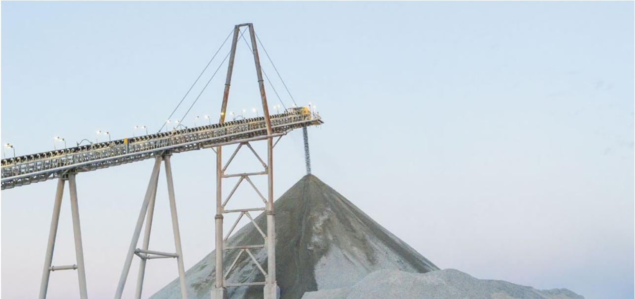
Image: Stockpile at the Pilgangoora Operation
